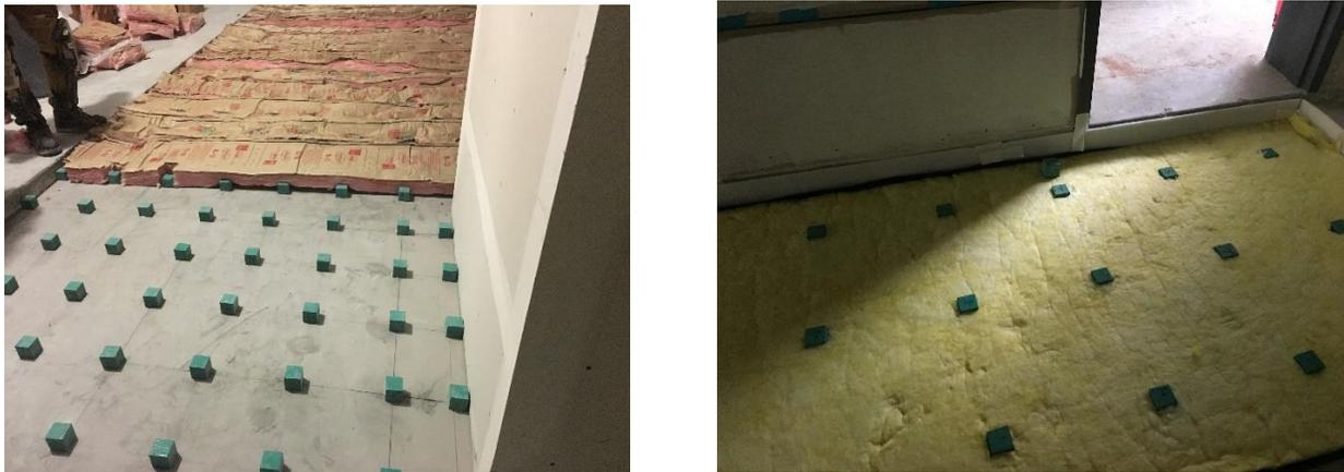
**Figure 8:** The installed floor (left) compared to specified product (right).
